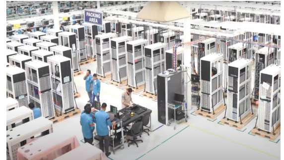
Rack Integration in Brno CZ Factory
