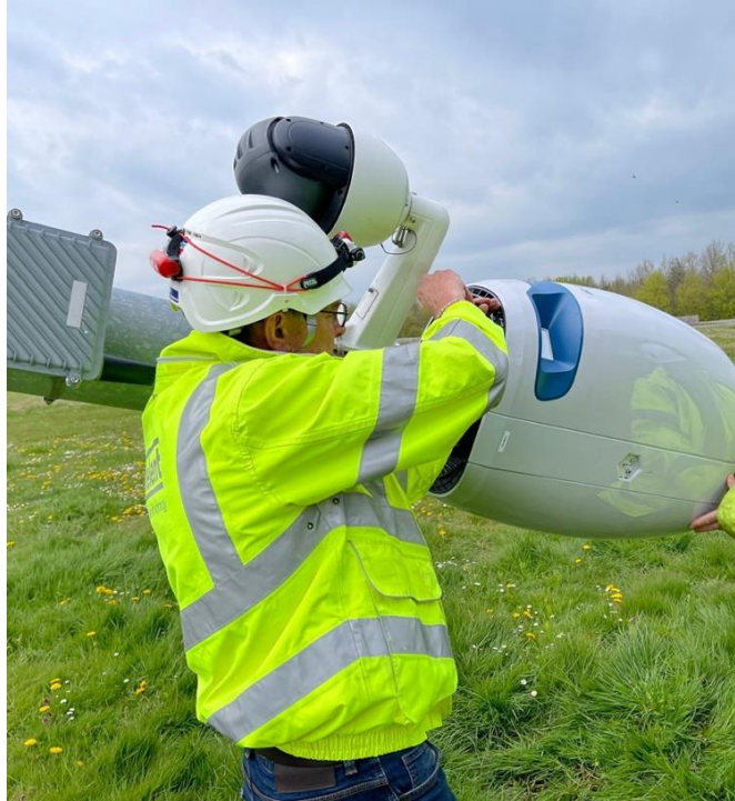
Figure 11 - Single CoMP-O-RAN unit installation on a winched pole
