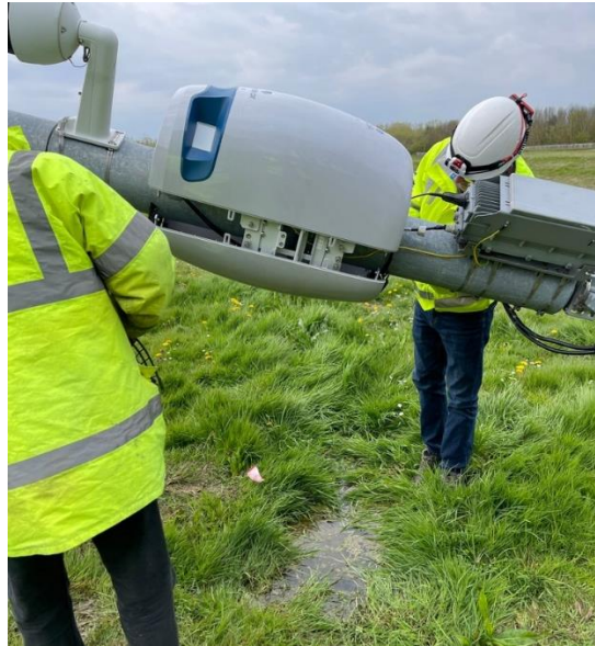
Figure 13 - Operational checks before repositioning the pole
