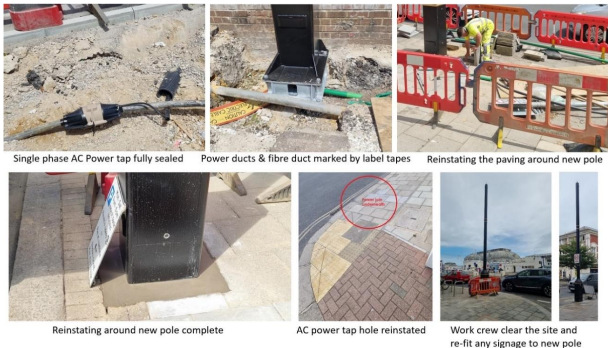
Figure 6 - Completing the ducting and re-instating the pavements
