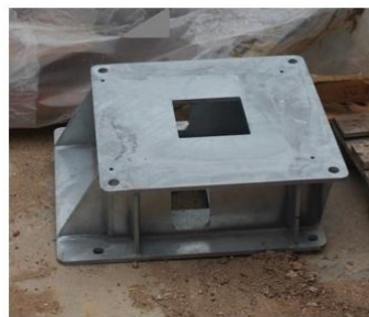
Offset mounting plate (upside down) Bolted into place on BFM once the concrete has cured (approx. 7 days)
