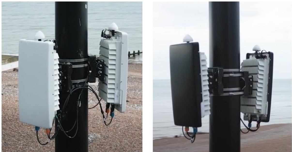
Figure 11 - Close up comparison view of the 5G radio assemblies before and after fitting black camouflage antenna panels
