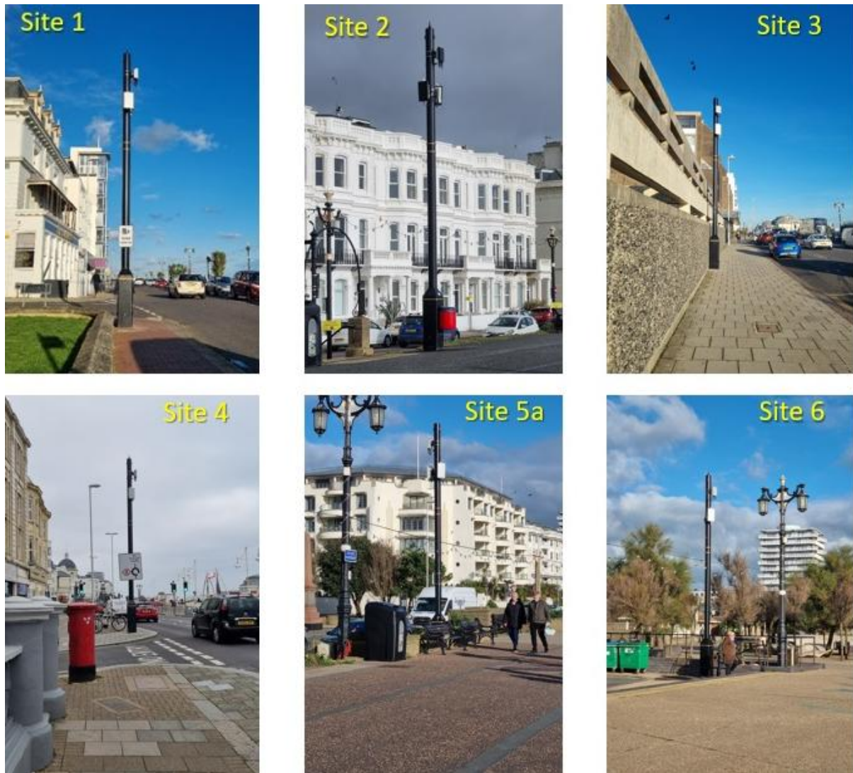
Figure 9 - Completed pole sites with 5G radios (also with 4G radios)
