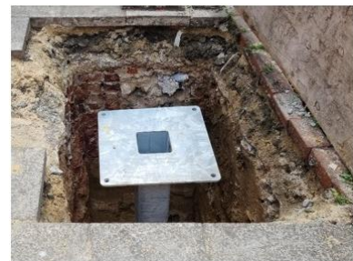
BFM on gravel bed in foundation hole
