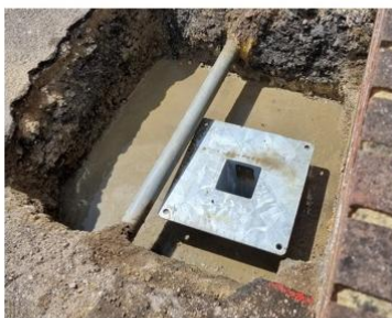
Foundation hole filled with concrete
