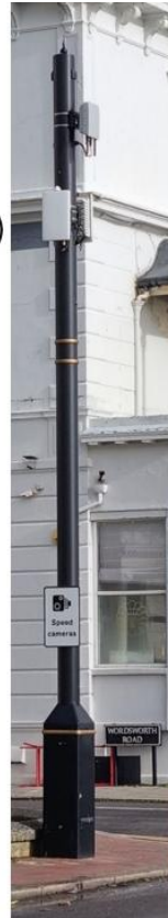
Figure 12 - Comparison view of poles with and without antenna camouflage as seen from street level
