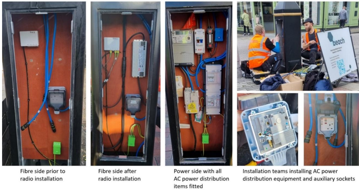
Figure 7 - Pole base preparations and electrical testing
